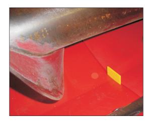
STEP 14 Wedge the panels tight against the bottom of the trough with the wooden shims supplied.
